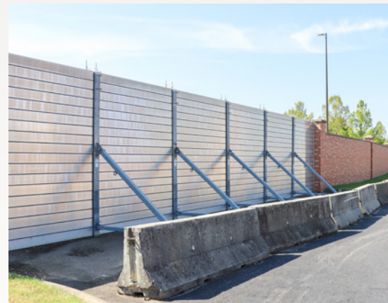
Gaylord Opryland Flood Wall
